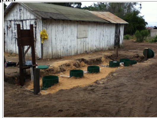
Completed installation before final backfill
