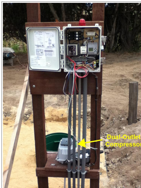
AquaKlear control center with AK Dual-Outlet Compressor
