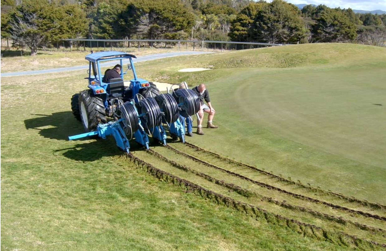
Photograph 2: Installing four lines at a time.
